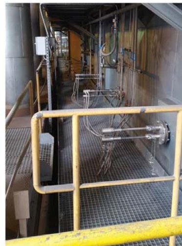
Injection lances for reagent and selective cooling
