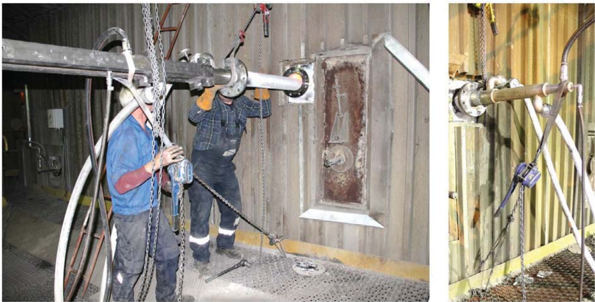
Figure 14: Installation of in-furnace lances for trial operation
