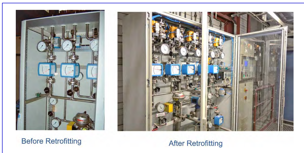
Figure 7: Control cabinet of an SNCR in a W-t-E plant retrofitted for \text{NO}_x < 150 \text{ mg/Nm}^3
