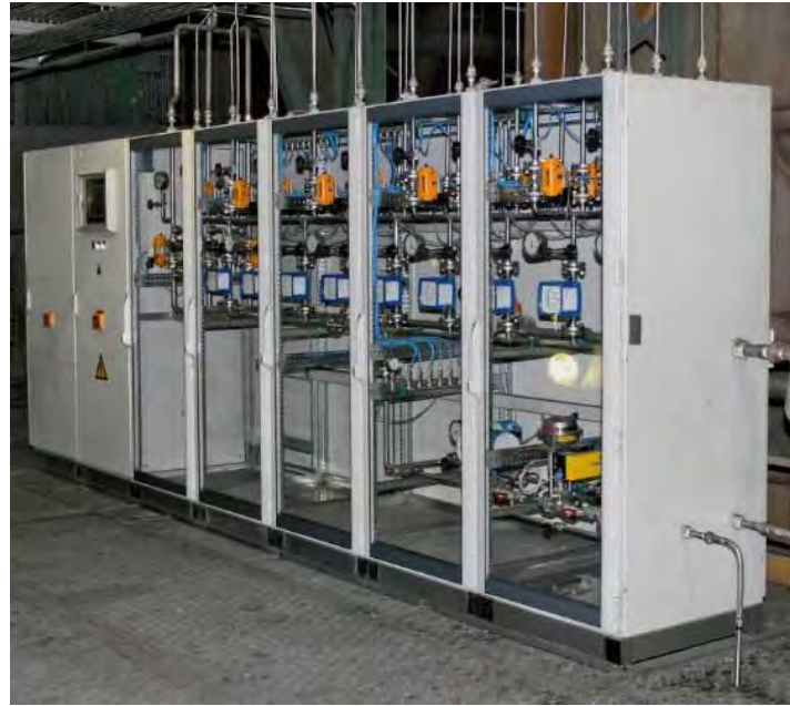
Mixing and metering module for SNCR in Jaworzno
