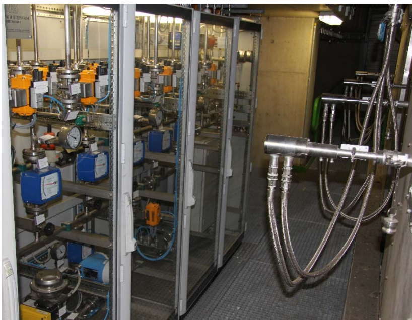
Figure 8: Mixing and Metering Module and Injection Lances
