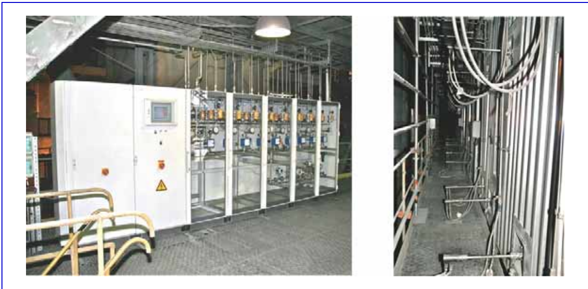
Figure 21: Jaworzno III - Mixing and metering modules and injection lances
