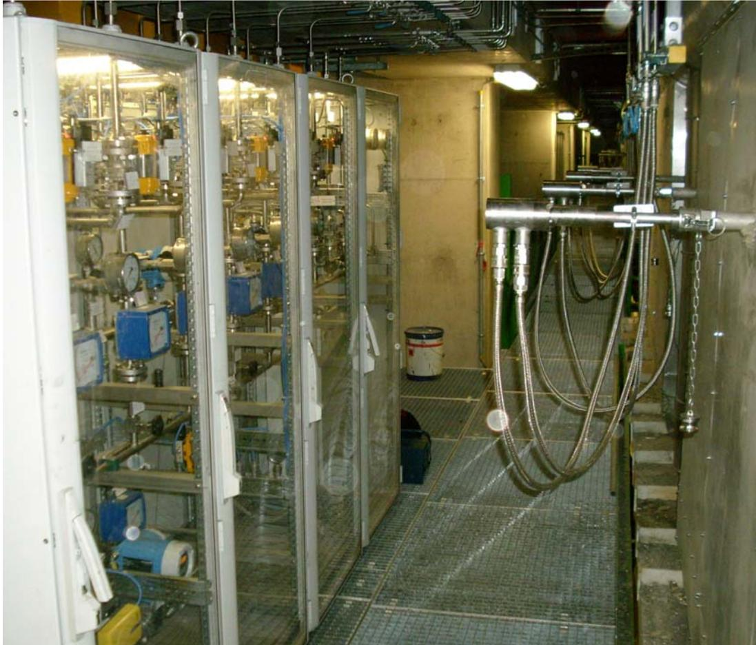
**Figure 8: Mixing and Metering Module and Injection Lances**
