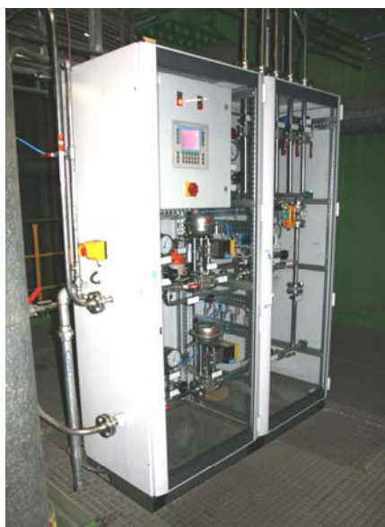
Fig. 7: Mixing and Metering Module - Distribution Module
