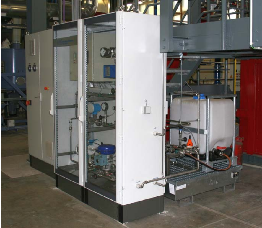
Fig. 2: Mixing and Metering Module and Container for Urea Solution
