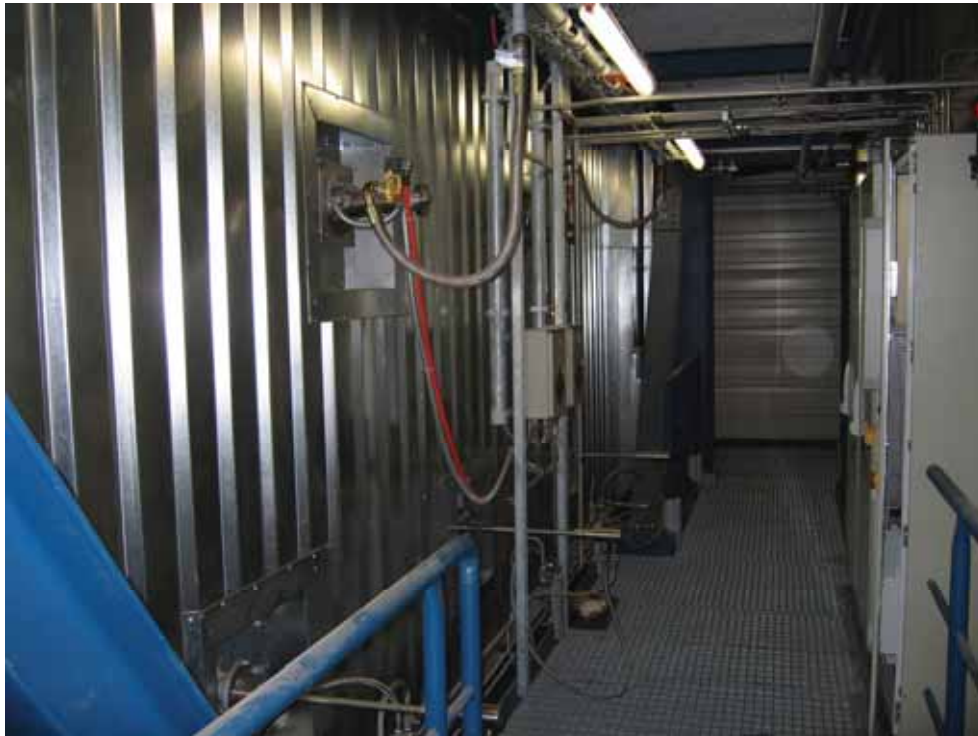
Fig. 8: SNCR Injection Lances with agam
